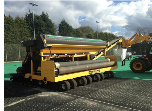
Automatic carpet lifting and rolling operation
