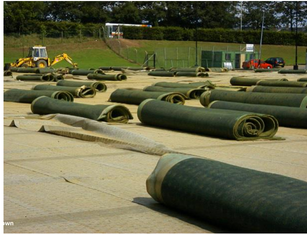
Rolled carpet ready for removal
